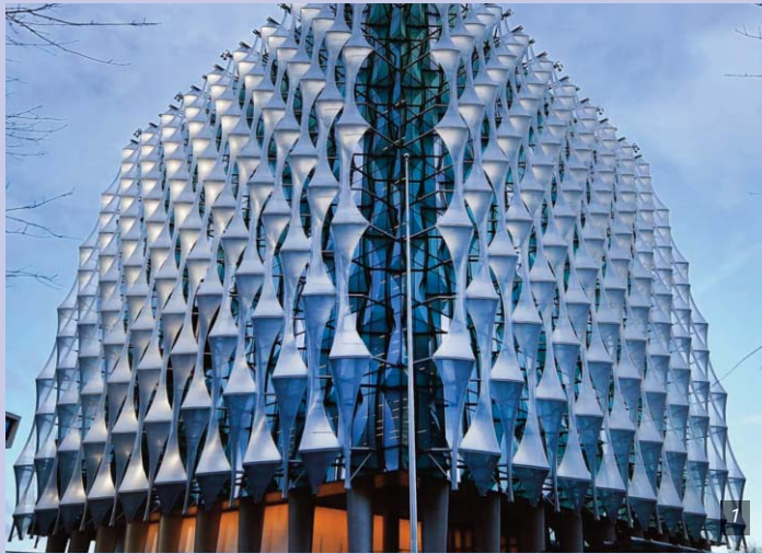
Figure 1. View on the US Embassy in London © BIRDAIR / Figure 2/3. Views on the membrane façade made of single-layer ETFE-sails © BIRDAIR
